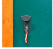
8. From the front of the door turn the key anti-clockwise to approximately 1 o'clock until the lock barrel is loose.
