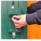
14. Replace the inner handle, fit the locking nut but do not over-tighten.
