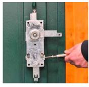
11. Replace the pozi headed bolt which locks in the lock barrel, this must be correctly aligned to engage in the lock barrel, do not over tighten.
