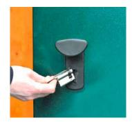
10. Push the new lock back into the door until it is fully located.
