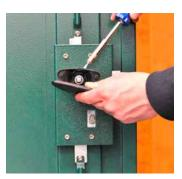
2. Remove the inner handle cover plate using a small slotted screwdriver and prise off the internal cover.
