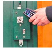
5. Using a 4mm allen key, remove the 4 bolts. Remove one pozi headed bolt from the centre of the lock cover plate.
