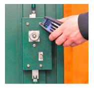
13. Tighten up the 4mm allen key bolts, ensuring that the pozi head screw is used in the centre of the plate.
