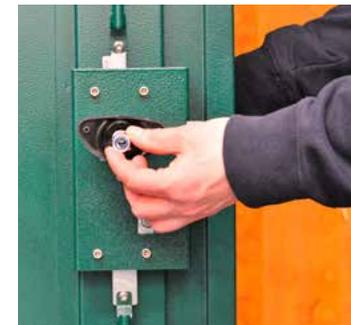
14. Replace the inner handle, fit the locking nut but do not over-tighten.
