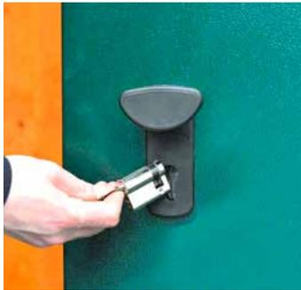
10. Push the new lock back into the door until it is fully located.
