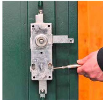
11. Replace the pozi headed bolt which locks in the lock barrel, this must be correctly aligned to engage in the lock barrel, do not over tighten.
