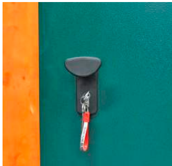
8. From the front of the door turn the key anti-clockwise to approximately 1 o'clock until the lock barrel is loose.
