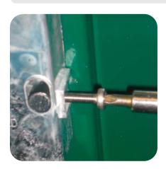
9. Replace the lock plate as shown ensuring that the pozi head screw is used in the centre of the plate.
