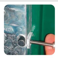
5. From the front of the door turn the key anti-clockwise to approximately five to twelve until the lock barrel be comes loose. Carefully draw the key back words, the barrel should slide out from the door, still attached to the key.
