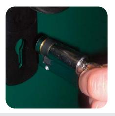
6. Push the key into the replacement lock barrel and turn it to approximately five to twelve so that the lock latch on the barrel sits flush with it.
